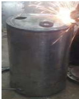
Fig. 3 Welding of Digester Tank
